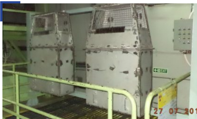
PCRDs installed at KAPS-1&2
