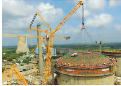
Erection of Dome Structure of Inner Containment at KAPP-3
