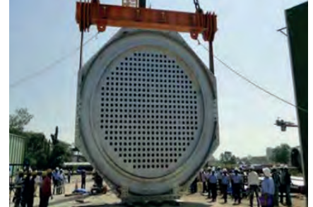
700 MWe End Shield received at KAPP-3, 4 Site
