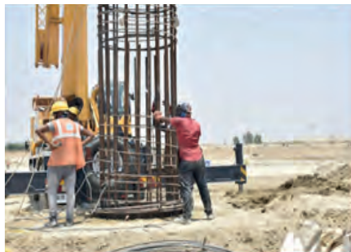
Head preparation for anchor piles in progress
