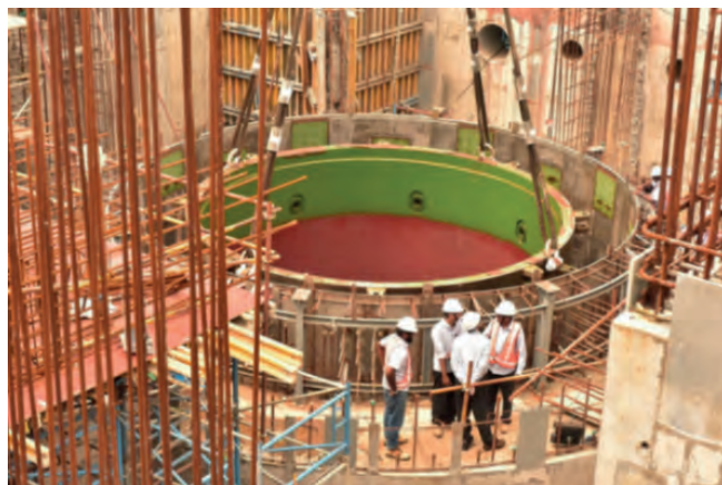
Core Catcher erection in KKNPP-3
