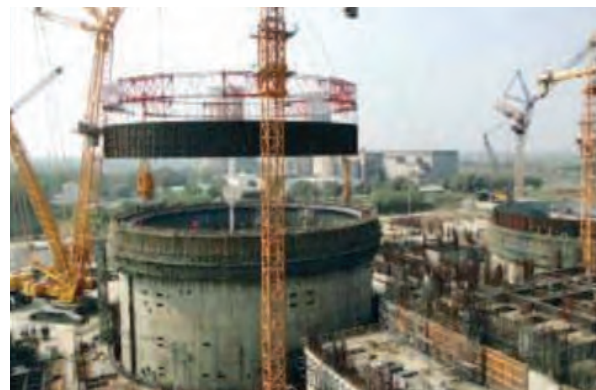
Installation of Pre-Fabricated Ring Liner at KAPP-3
